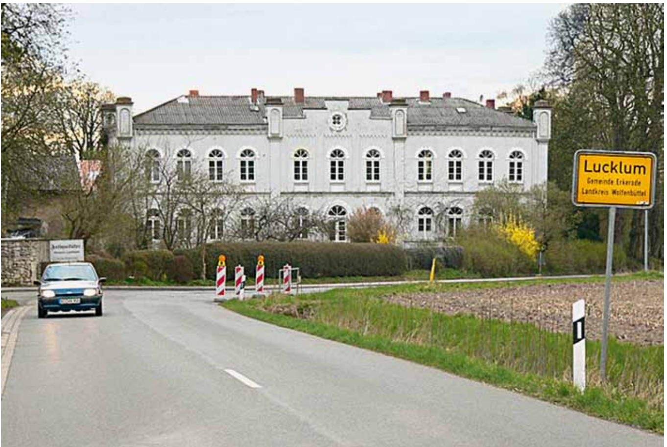
1 Entrance to Lucklum in Lower Saxony
