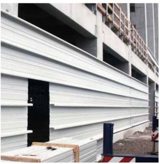
Façade fixed using HALFEN HTU Cast-in channels
