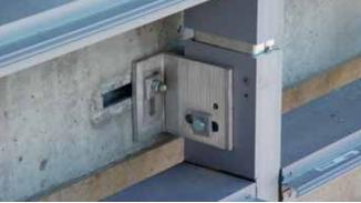
Fixing of a post and beam façade using HCW-ED brackets on HTA-CE channels
