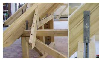
Timber roof construction with HALFEN HNA Fixing straps
