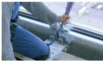
Fixing of a modular façade using HCW-ED brackets on HTA-CE channels
