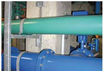
Pipe supports on vertical HZA-channels
