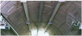
Curved HALFEN Cast-in channels in tunnel segments
