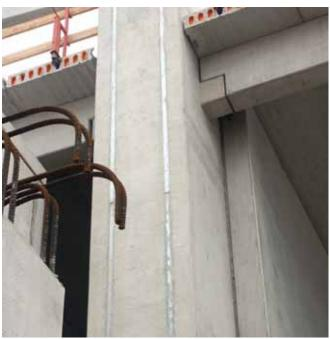
Vertical HALFEN HTU Cast-in channels for connecting façade panels
