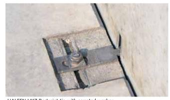
HALFEN HKZ Restraint tie with serrated washer
