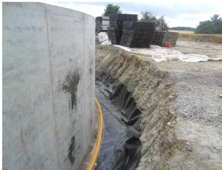
Installation: foil – drain fleece - drain tube
