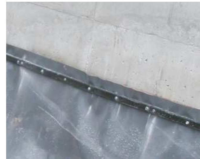
control tube – fixing the foil at the concrete tank
