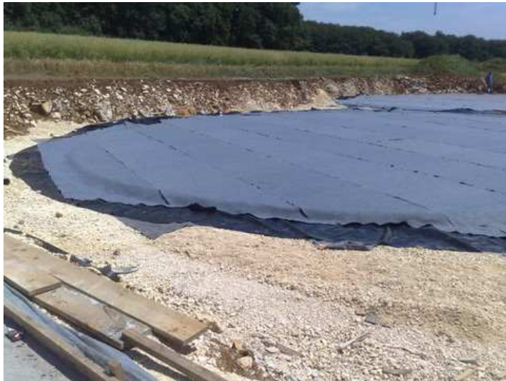
Installation: foil – drain fleece - drain tube
