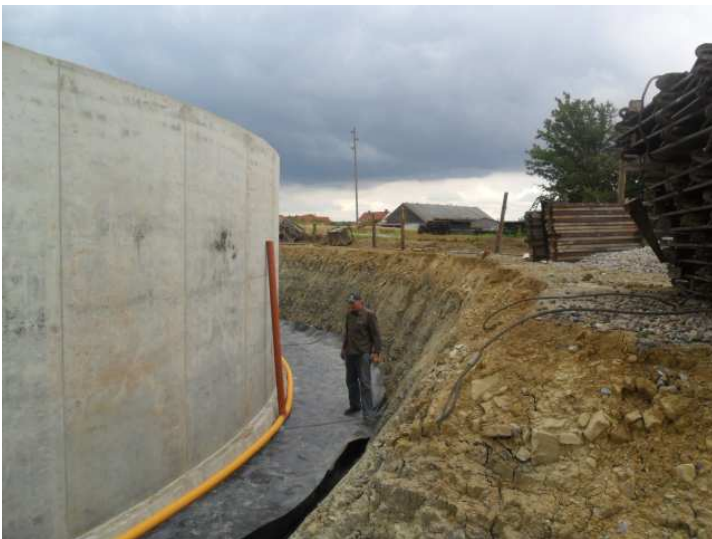
control tube – fixing the foil at the concrete tank
