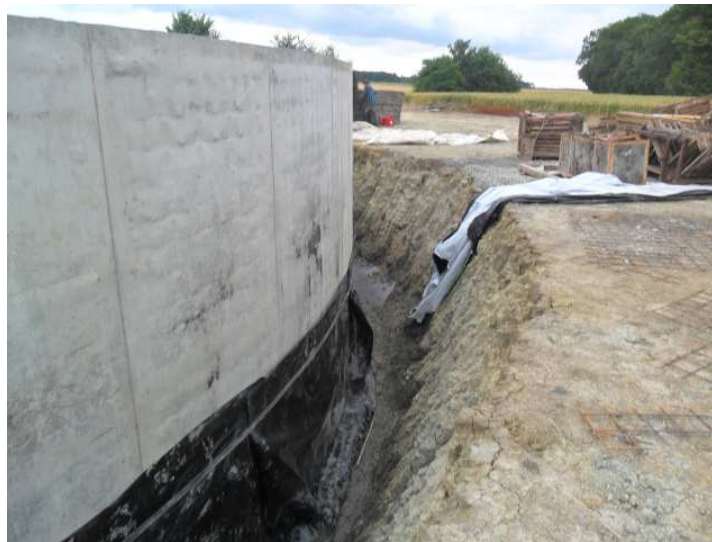
control tube – fixing the foil at the concrete tank
