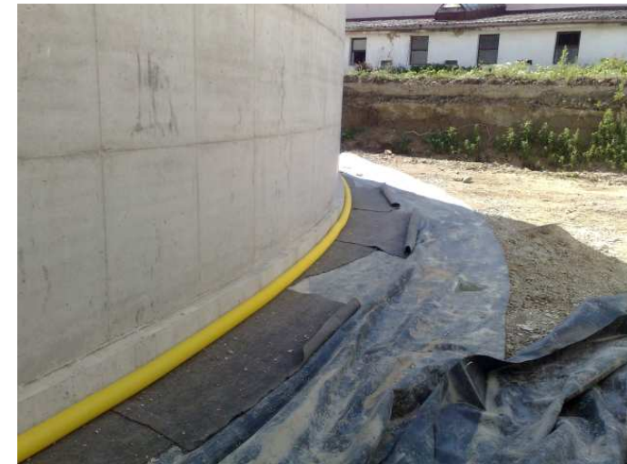
Installation: foil – drain fleece - drain tube
