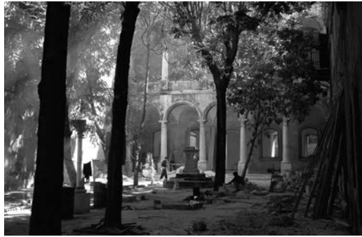
Restoration of the Shibani building
