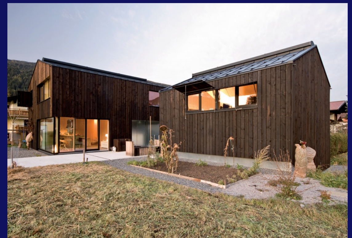
LP architektur Haus Trattner-Scharfetter, Radstadt, 2010
