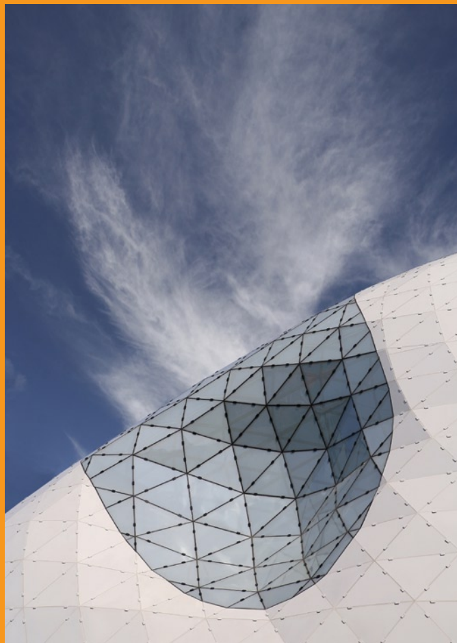
Massimiliano Fuksas architetto Blob, NL-Eindhoven, 2009 Turn On Partner: Waagner-Biro Stahlbau AG Foto: Rob Hoekstra
