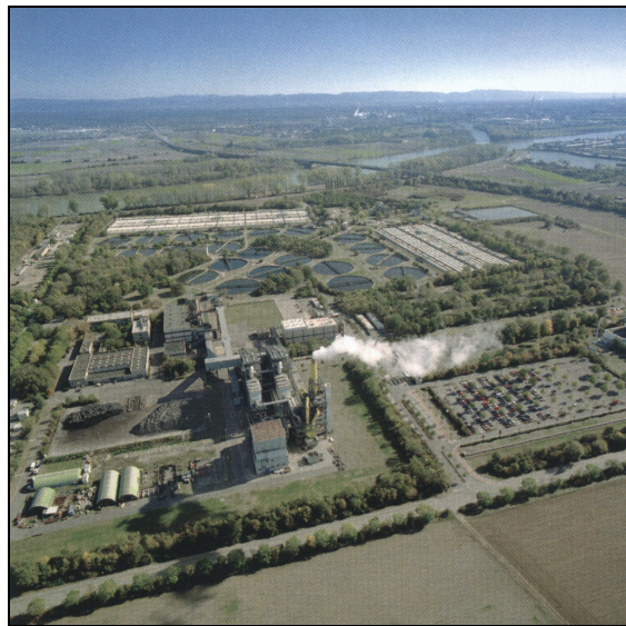
Figure 19 Sewage works at BASF factory in Ludwigshafen (source: BASF)
