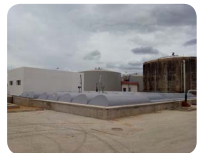
Example: Sewage treatment plant Badajoz / ES with BIOMOX® CFR
