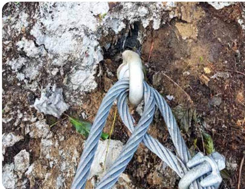
Figure 1: Examples of the use of micropiles for protective structures; lower foundation (above); rope anchor point of a step-down transformer on the hillside (below)
