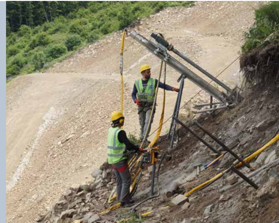
Figure 7: Drilling for stabilisation works along the detachment zone of the rockslide
