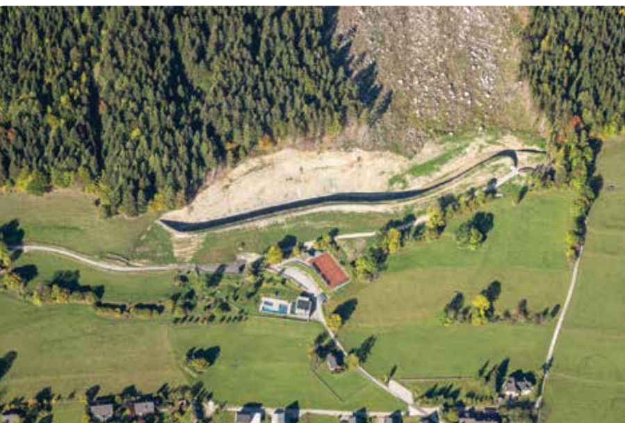
Figure 8: Completed rock fall protection dam
