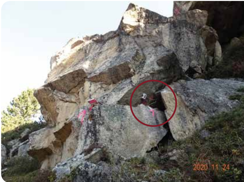
Figure 6: above: Fissurometer (yellow rectangles) and below: reflectors (red circle)
