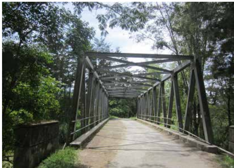
Road and bridge in Jayawijaya, Papua, Indonesia, 2021
